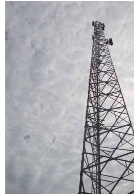
Figure 24: Tanzania/ A new 3G tower built by Vodacom in the middle of the Nyarugusu camp, Tanzania
