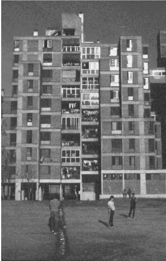
Photograph 2: Public rental housing in Buenos Aires, Argentina
